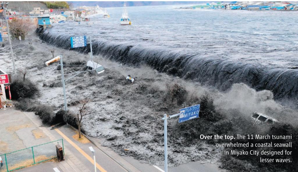
Over the top. The 11 March tsunami overwhelmed a coastal seawall in Miyako City designed for lesser waves.
